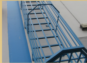
Roof Access Ladders
