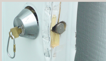
Emergency Door Repair
